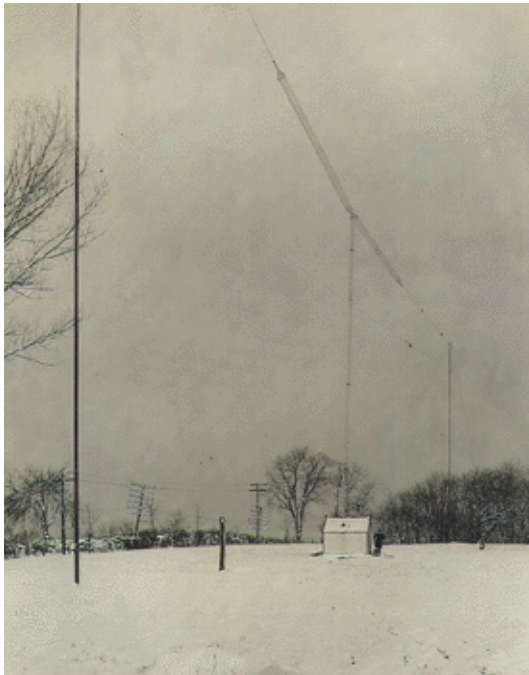
A 1921 view of 1BCG, located on a field of the Elisha P. Cronkhite estate in Greenwich, Connecticut. The flattop T cage antenna is supported between two steel masts 108 and 75 feet tall. This was the cover photo for February 1922 QST, and was also published in the Scientific American article (see sidebar) and in other reports of the event.
